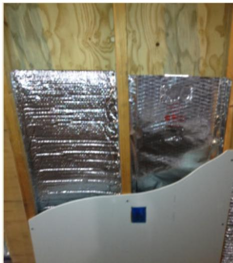
Figure 2. Reflective Insulation Installed in Floor and Wall Applications
